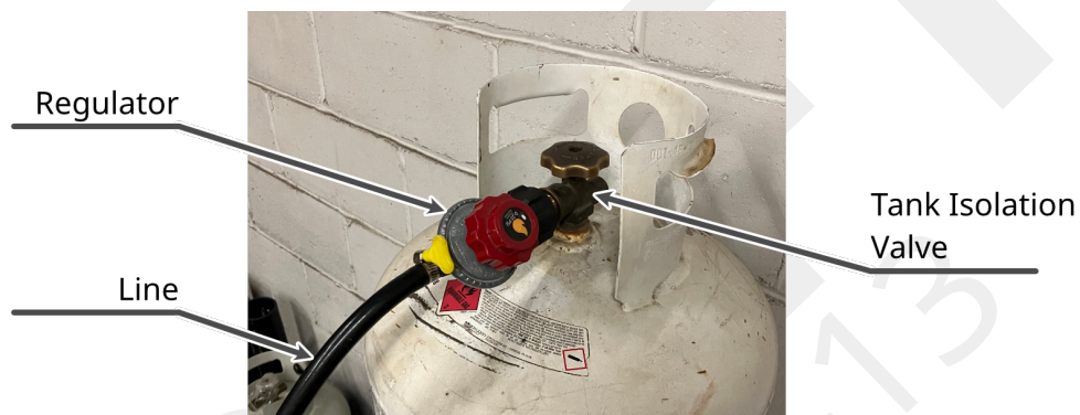
Figure 1: An annotated view of the large propane tank.
